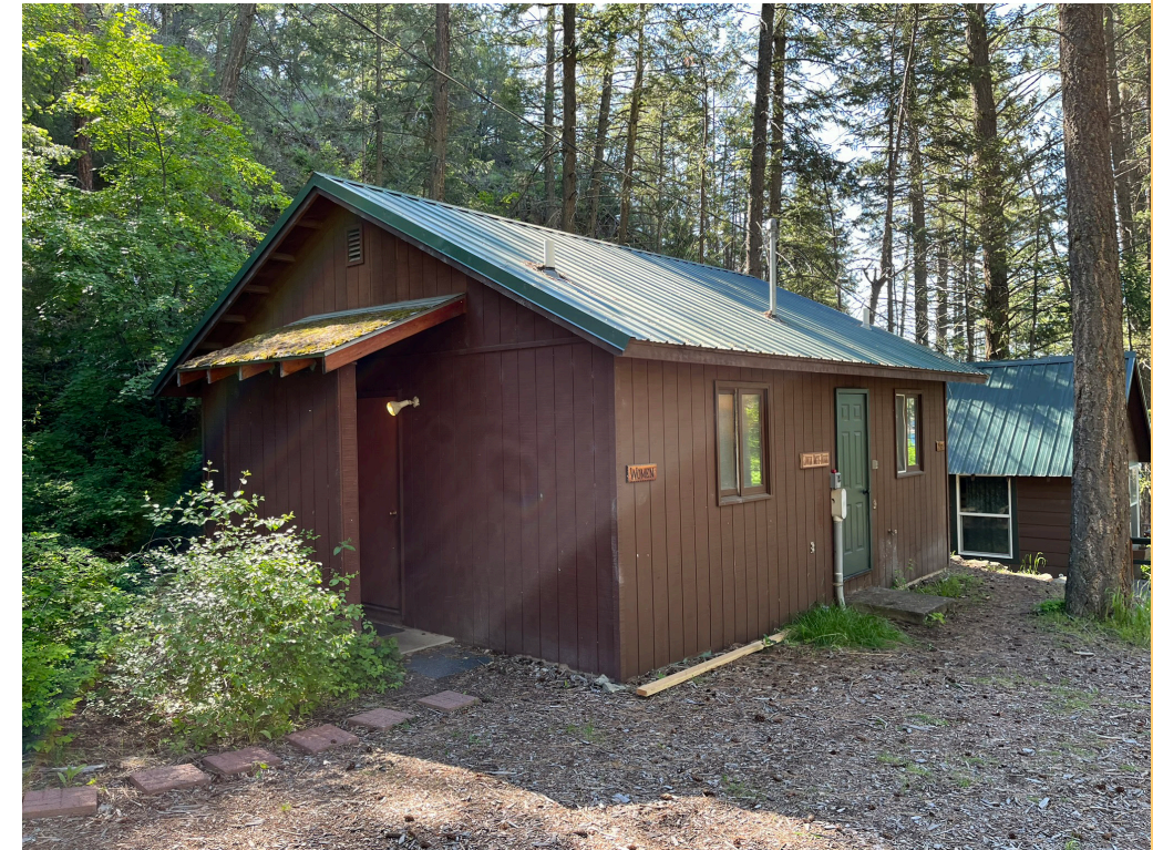
G3 East Bathhouse
